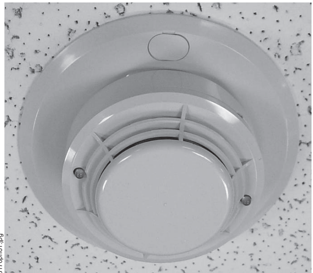
B501BH shown with a smoke detector
